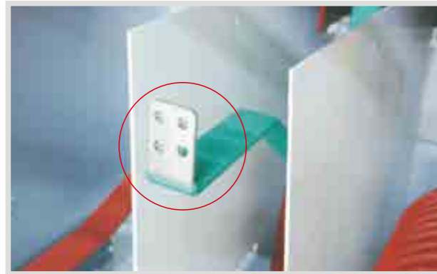
Tinning, leading angle, deburring and knurling at tap joint to all busbars, degrade the resistant of lap.
